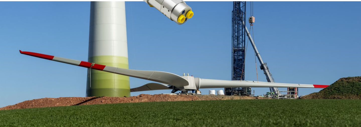
Tower and wing assembly for wind turbines
